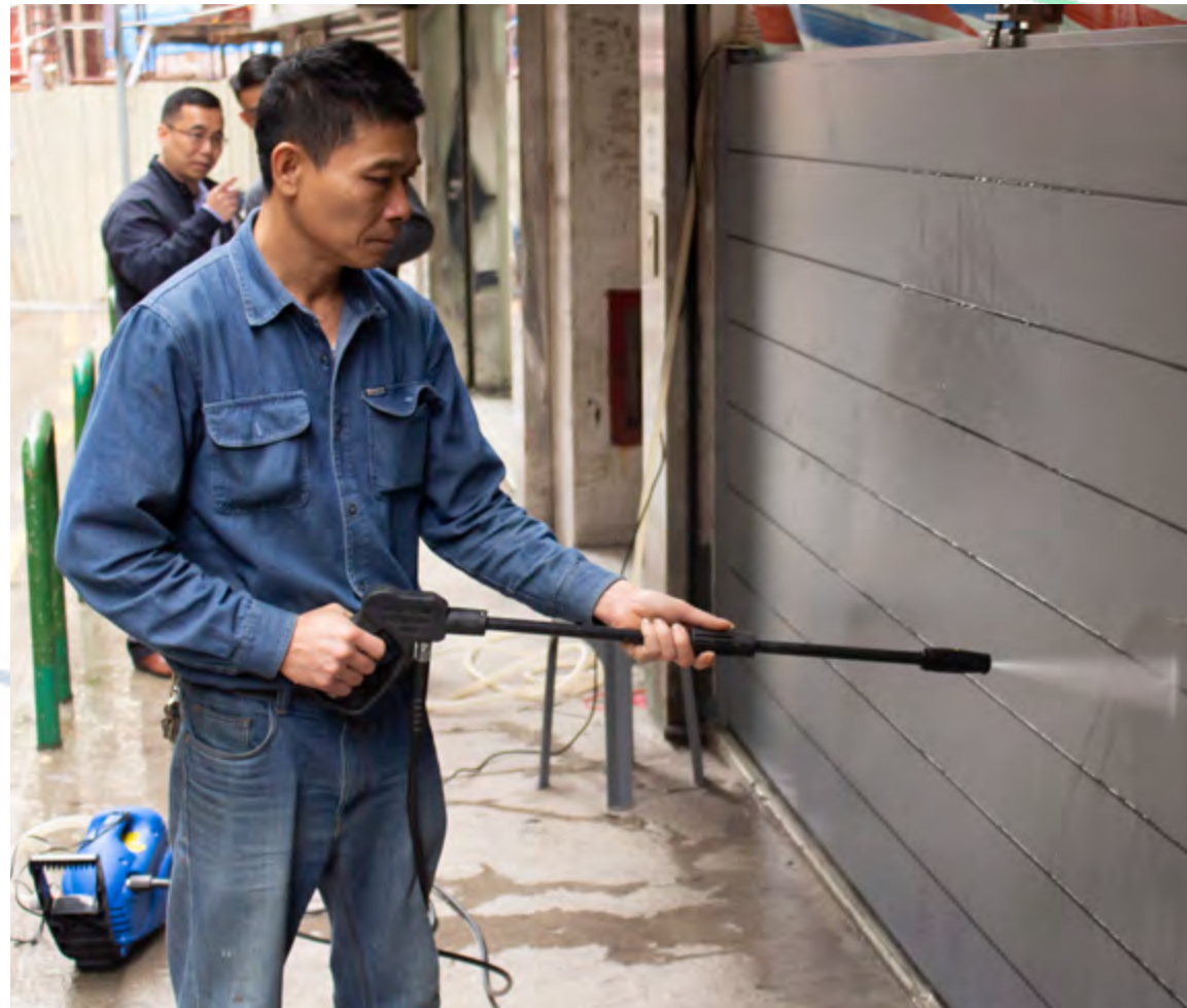
加強對防洪閘的水密測試 More water tightness tests were conducted on flood gates.
